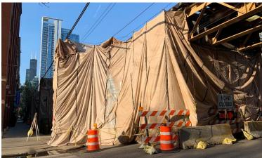
Preparation of the containment area and cleanup of the sandblasting for upcoming paint work
